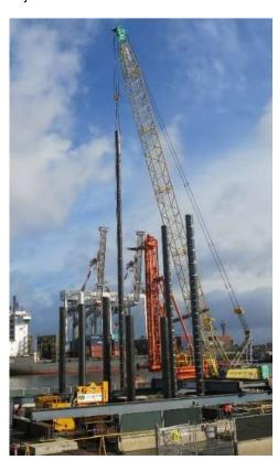
To rehabilitate the concrete fender beams, McConnell Dowell developed and engineered a fender access platform that provided a safe working platform across a 15m x 4m footprint. The platforms provided safe access from land to the front, soffit and rear faces of the fender beams, to allow hydrodemolition works, reinforcement replacement and augmentation, and shotcrete spraying of the fender beams.
