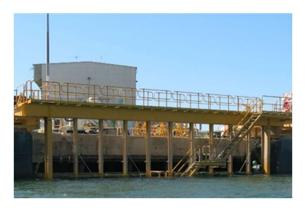
The reusable platforms were designed so all the elements of the works could be undertaken from a single set-up. The platform also included removable mid-level decks to provide safe access to the full fender depth and underside of the wharf.
